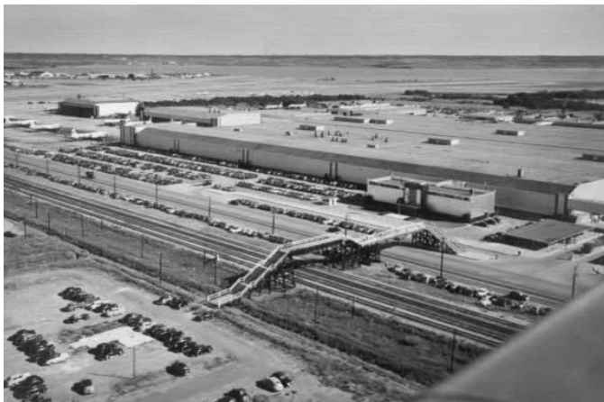
Pedestrian bridge over railroad tracks, from parking lots to flagpole entrance to JSF
